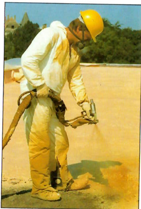
Jointless application of Baymer DS-1 spray-on roof foam is possible on any dry substrate
