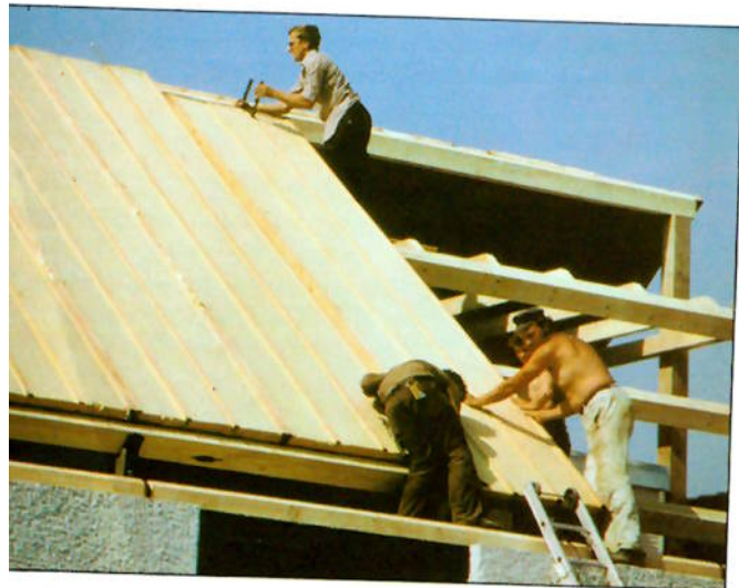
Self-supporting roof sections are laid on top of the purlin framework
