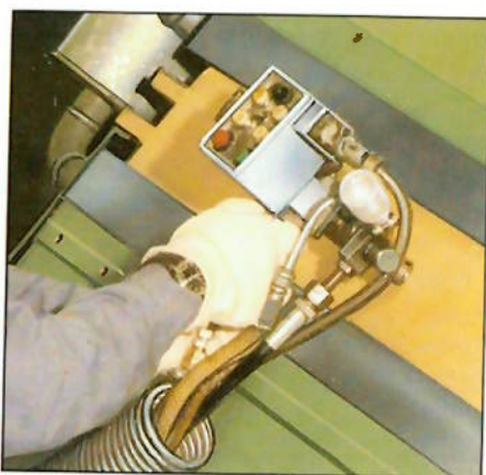
Filling a cavity with foam
