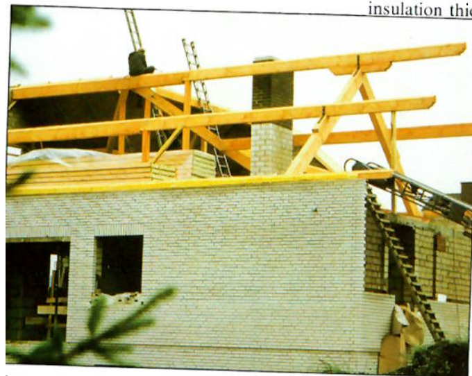
Fixing the purlin framework
