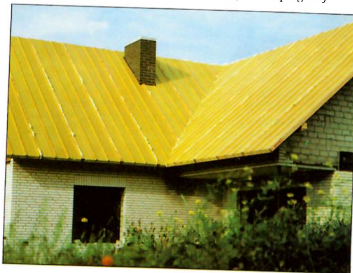
A steep-pitched roof with Baymer-insulated sandwich sections
