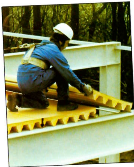
Fixing the light-weight sandwich section in place on steel joists
